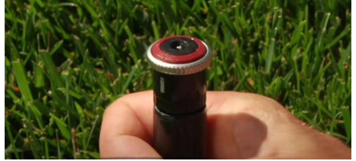
Rotate head to start arc from correct point
