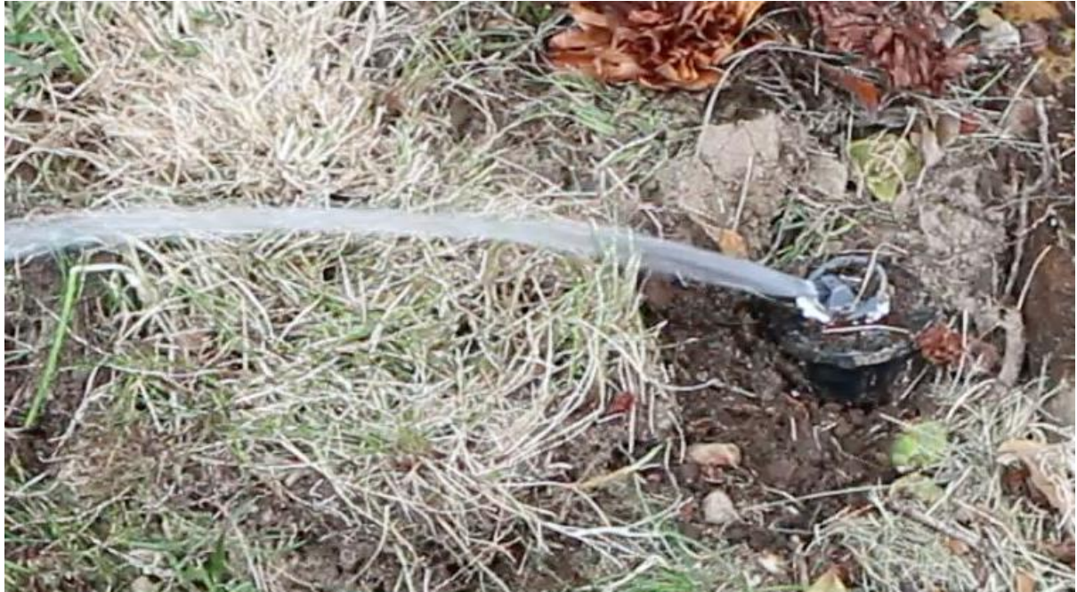
Flushing the system with the flushing cap still in place
