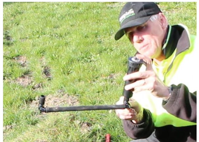
Connect Heads with Swing joints
