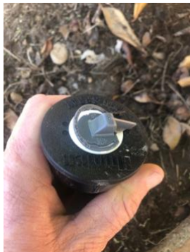
Flushing the system with the flushing cap still in place
