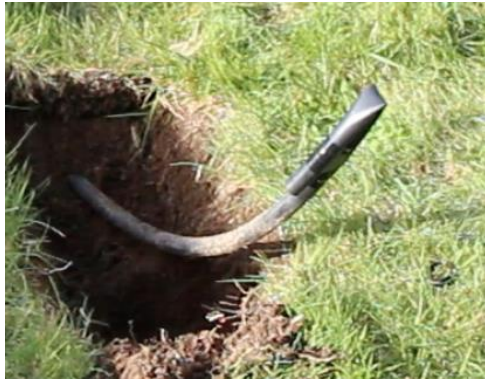
Pipe at sprinkler location
