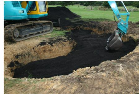
Fig.3 Soil mix placed to compact naturally.
