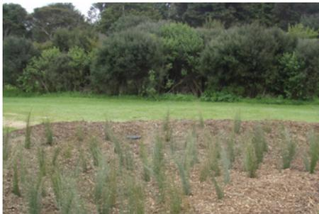
Fig.5 Finished rain garden, planted, with mulch layer
