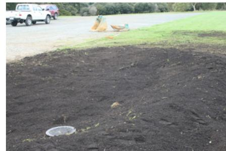
Fig.4 Soil contoured to form ponding area. Overflow structure is screened.
